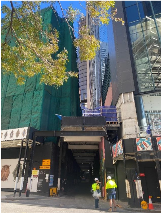
Figure 3: Existing gantry hoarding along Underwood Street (hoarding erected in association with Lend Lease development of 'Sales Force' tower immediately to the north of the site)
